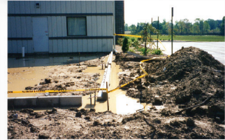
First building erected on 8363 Embury road.
